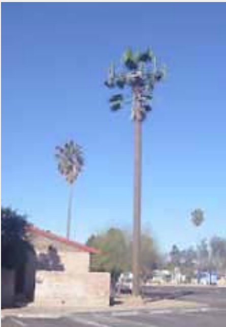
Camouflaged microwave tower, Tucson
