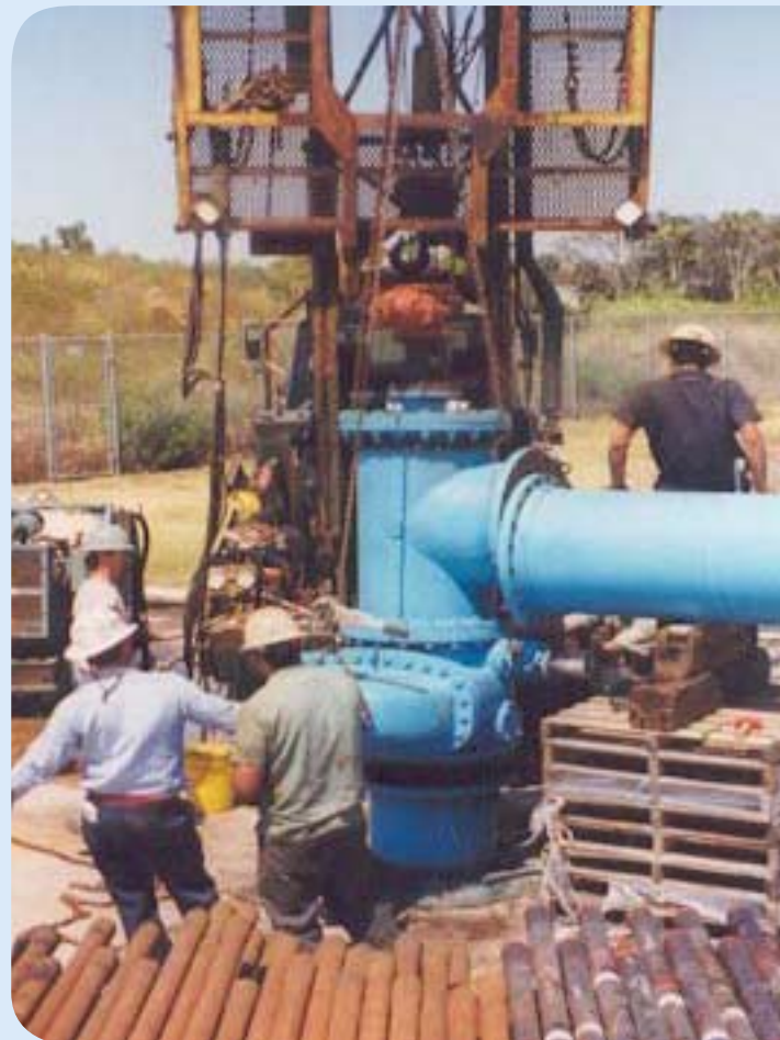
Figure 4: Workers at a Class 1 injection well
